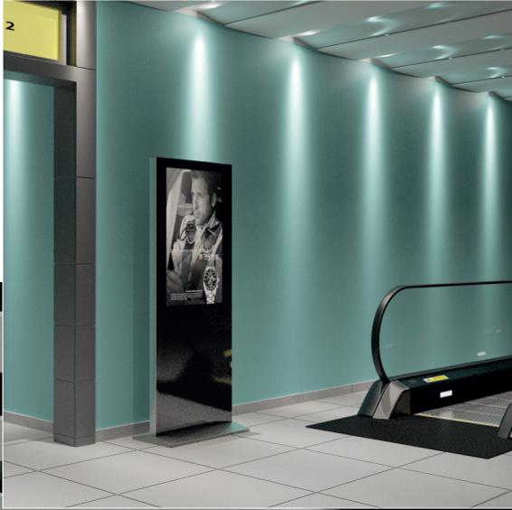
The linear wall emphasises the clean installation that Tongue & Groove, together with colour matched sealant provides. 'Return tile' upstands complete the finished appearance.
